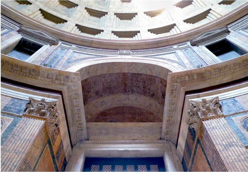
1. The barrel vault over the interior entrance alcove of the Pantheon, seen from below
